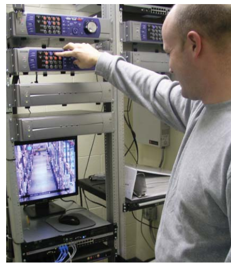
The Hawthorne Distribution Center is under 24-hour surveillance.
